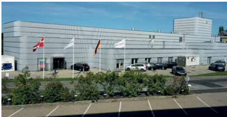
SPX FLOW Innovation Center in Soeborg
